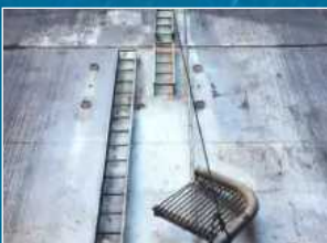
ON / OFF HIRE BUNKER & CONDITION SURVEY
